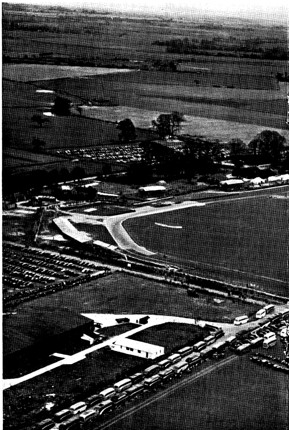
AERIAL VIEW OF GOODWOOD
