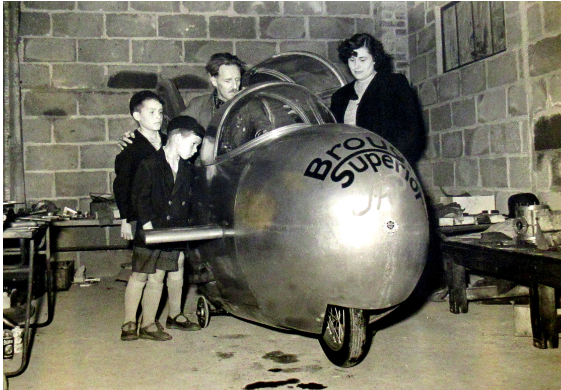
Figure 4. Noel Pope and family with the streamlined Brough Superior before the record attempt in September 1949, possibly taken in a workshop at Comerfords of Thames Ditton. Note the side fins that were intended to stabilize the machine at high speed. Computer-enhanced image of a photograph taken in the Brooklands Museum Library by David A. Kennedy.
