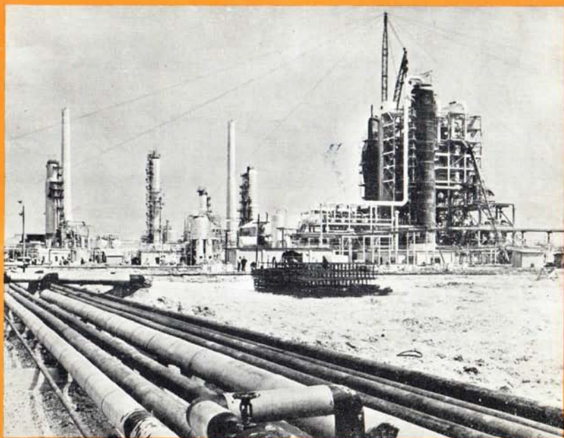
A Section of the NEW ESSO REFINERY at FAWLEY
